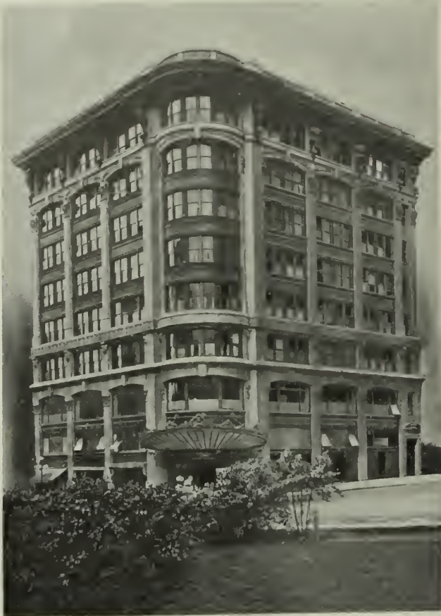
THE GUNST BUILDING. Lansburg & Joseph, Architects.
